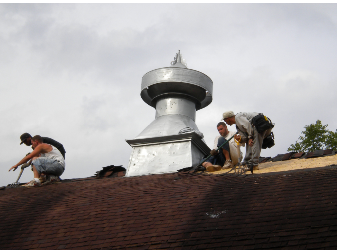
In August, thanks to funding from the CRST International Fund of The Greater Cedar Rapids Community Foundation, the 1932-era former dairy barn received a new roof.
