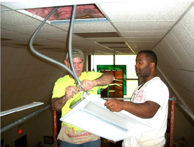
Electricians install new LED lights in the auditorium. Alliant Energy, Munson Electric, and Van Meter Inc provided conversion assistance to more efficient building lighting.
